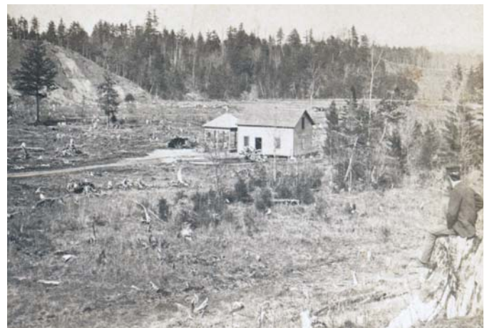
Figure 4. View of clear cut area, Champlain Spring, Highgate, Vermont, late 1800s. In the background are landslides on a steep, cleared slope. Field work suggests failures are in silty, fine sand, glacial lake deposits of the Champlain lowland. These shallow planar slides were likely catalyzed by loss of effective root strength after clear-cutting of the slope (see Fig. 3). In the middle ground are many stumps and much slash, the remains of cutting second-growth timber. There is a spring house at the center of the image. Note the tremendous size of the stump on which the man is sitting; it is likely all that remains of the old growth, pre-settlement forest that once covered Vermont lowlands like this. Image property of University of Vermont, Special Collections, Bailey Howe Library (LS03668).
