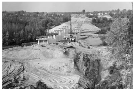
Figure 3D. Same view as 3C, during interstate construction in October, 1961. Note scale of disturbance and riparian changes.
