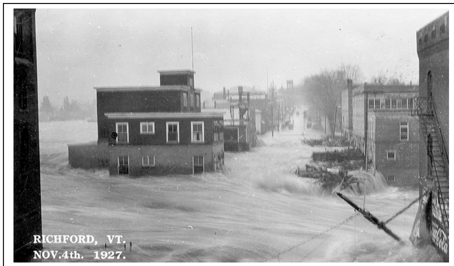
Figure 6. Image of the 1927 flood inundating Main Street in Richford, Vermont. From University of Vermont, Bailey Howe library, Special Collections.
