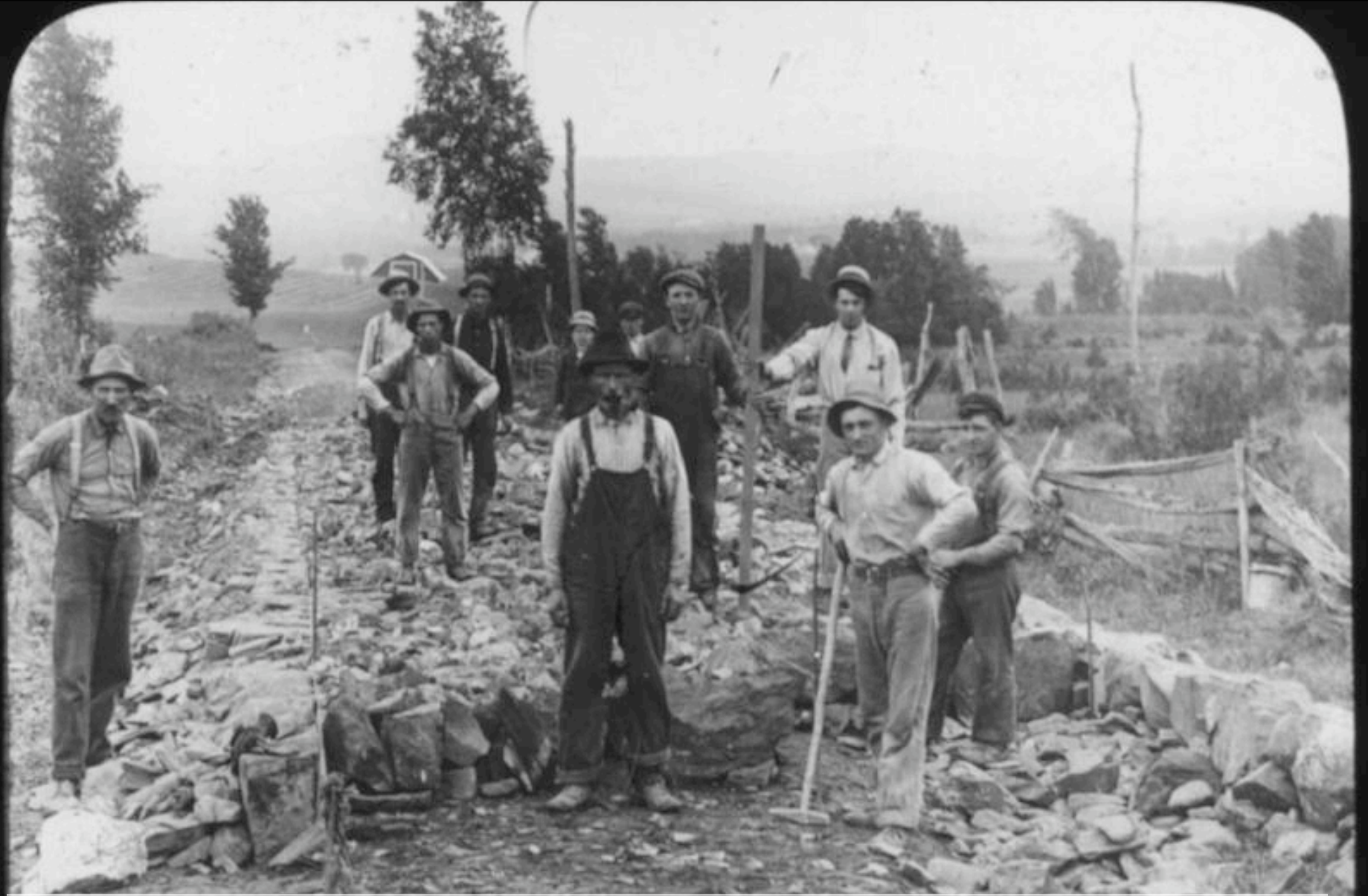
The title on the photograph was "Telford Foundation". Lanternslide.
