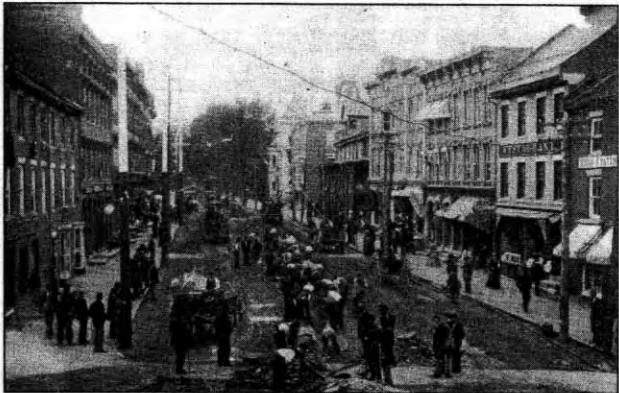
State Street, during the installation of trolley tracks, late 1890s. Here we see utility poles crossing over the street, and the thick canopy of State Street's elms in the distance. UVM Landscape Change Program. LS05638: Vermont State Archives.
