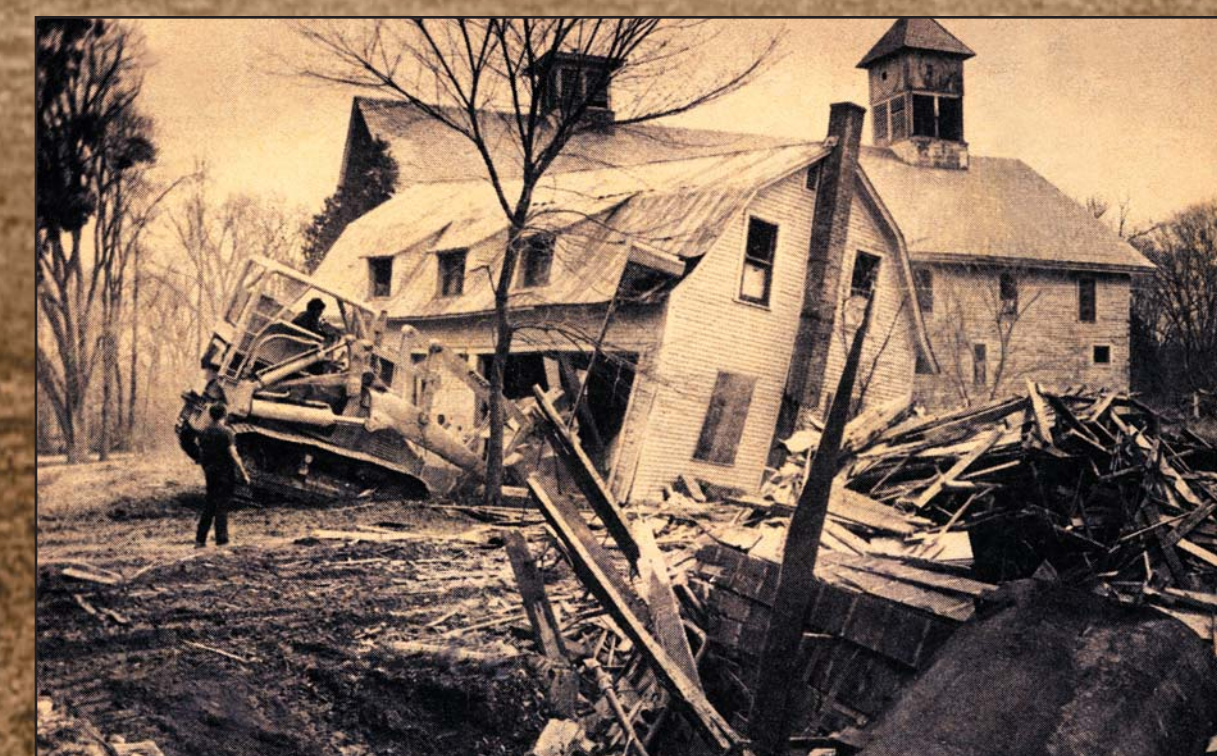
After many years of use, the barn and garage gave way to bulldozers in May 1975, making space for the Ledgewood development.
