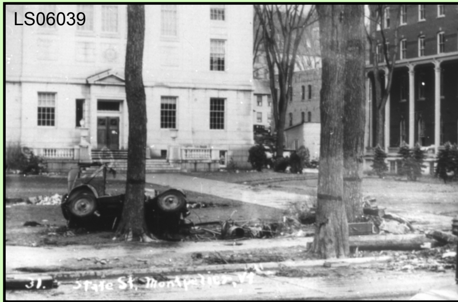
Montpelier, 1927. Photo shows flood damage at state capitol. Note variation in color on tree trunks indicating height of flood waters
