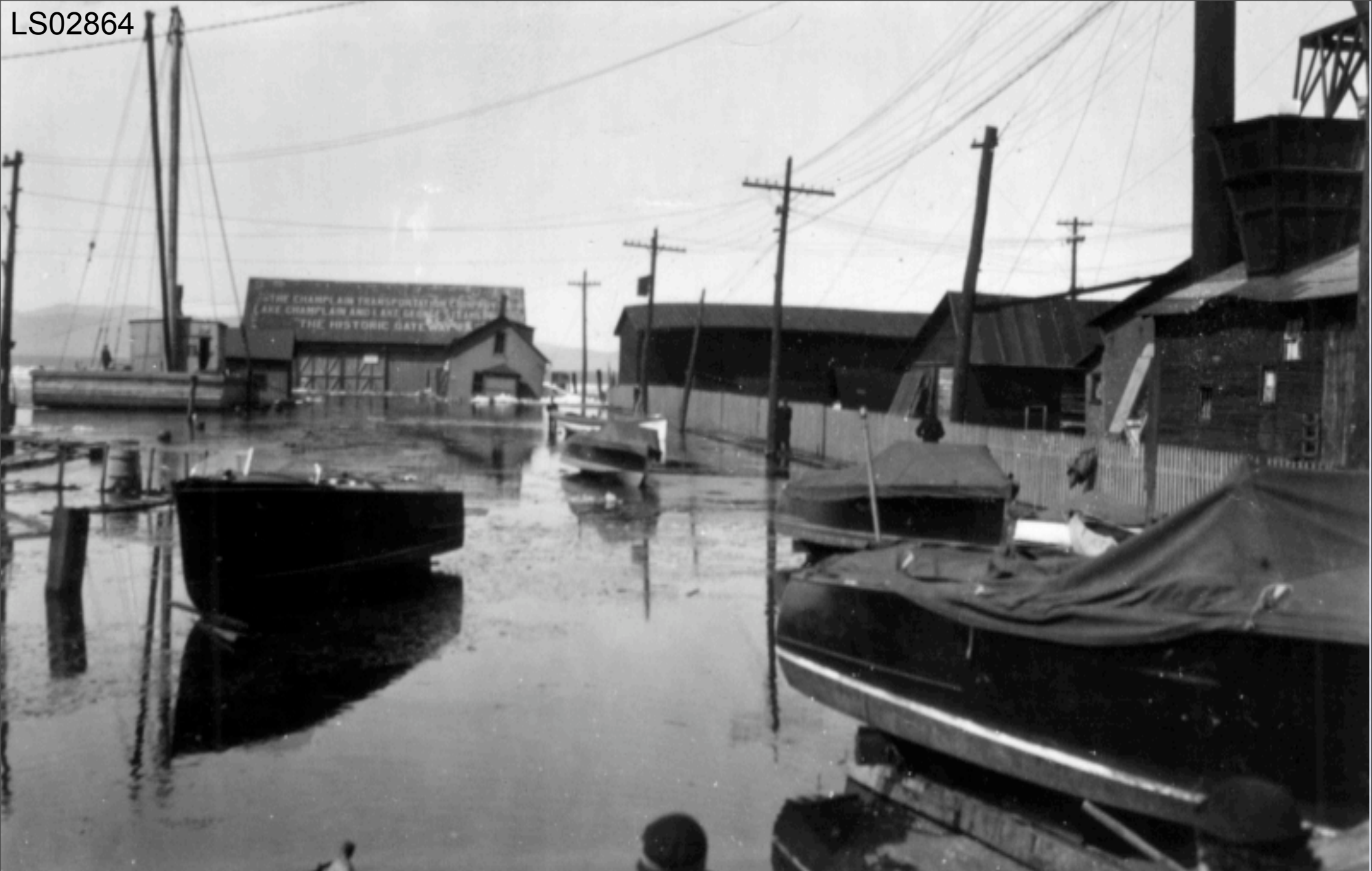
The Champlain Transportation Company has been running ferries across the lake since the 1840s. Obviously, they've had some troubles along the way. This is the King Street Ferry dock in 1936, after a spring flood washed a number of boats onto the road, probably from the adjacent Perkins Pier marina.
