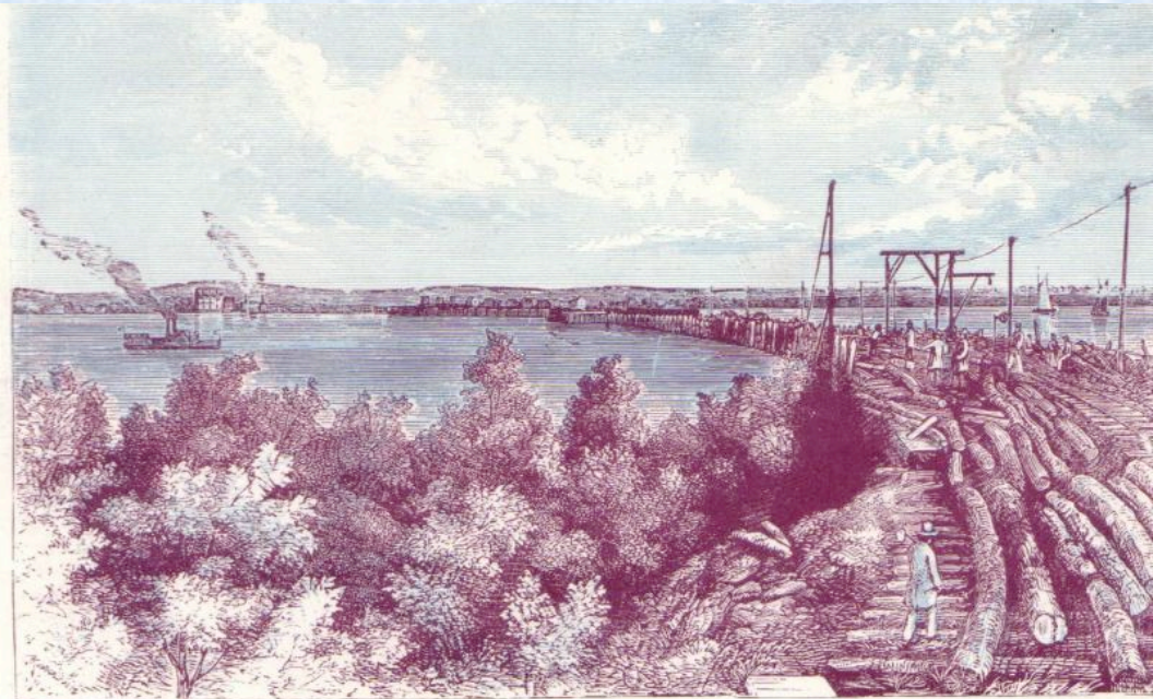
R. R. BRIDGE, AT ROUSE'S POINT.
