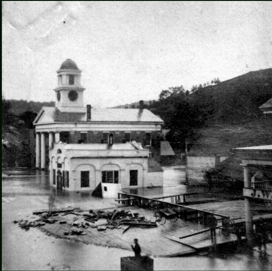
FLOODED COURTHOUSE AND BANK ( 1869-10-04 EXACTLY ) LS03906_000
