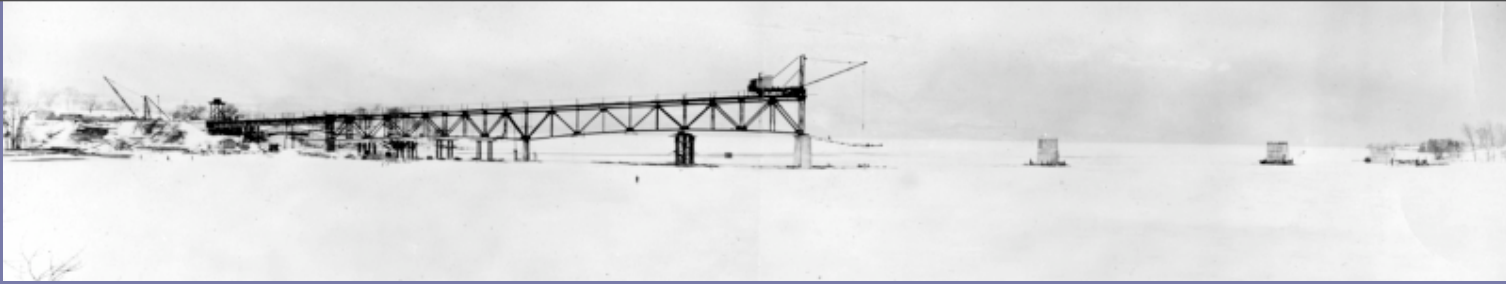
This image shows the construction of the Champlain Bridge in Addison, VT 1929. LS06711
