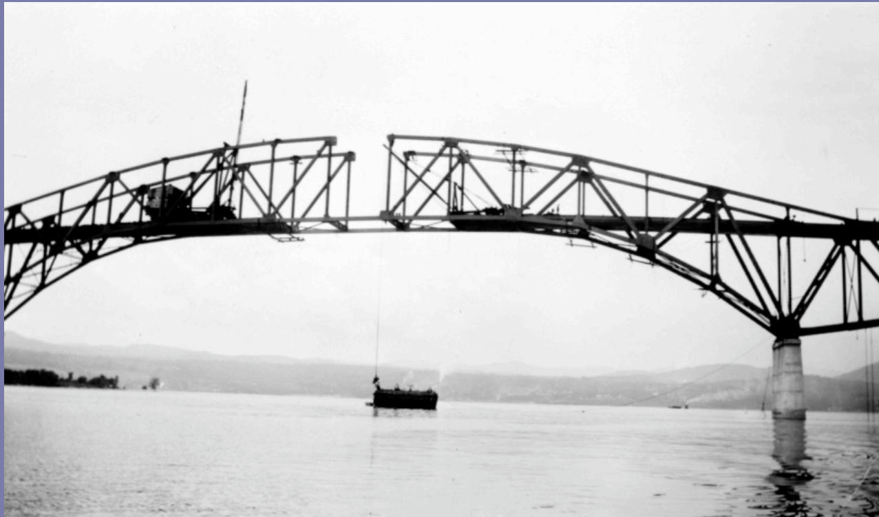
Passenger steamers declined with the construction of bridges which crossed the lake and introduction of the automobile to the region. The photo above also displays the construction of the Champlain Bridge in Addison, VT 1929. LS06713
