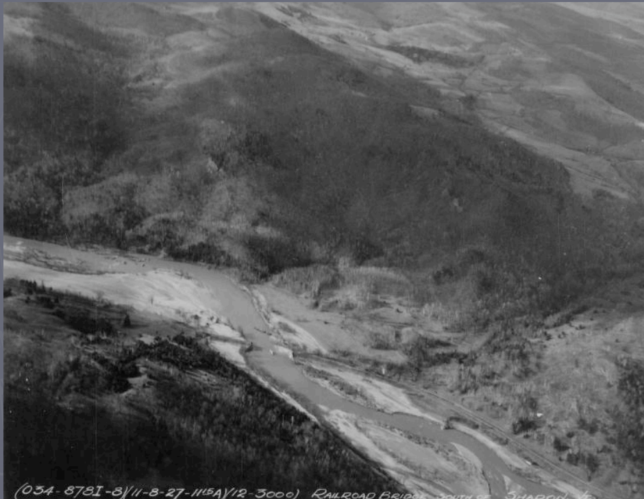
(05A-878I-8/11-8-27-1115A/12-3000) RAILROAD BRIDGE SOUTH OF SHARON, VT.
