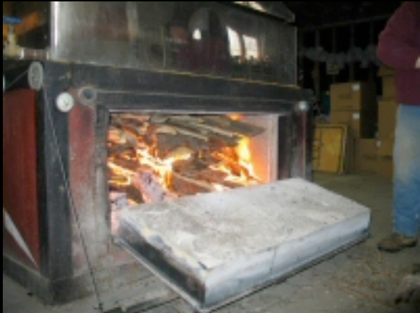
Bottom of Evaporator
