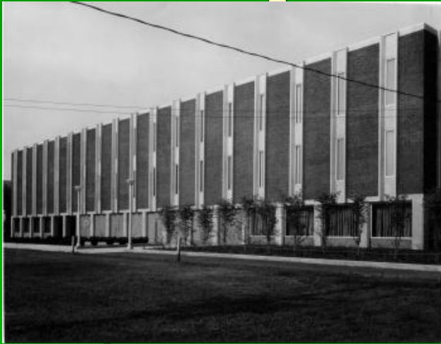
Votey Building is the Math and Engineering Department's home, completed in 1962.
