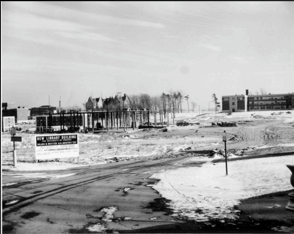
Bailey Howe Library Winter Construction
